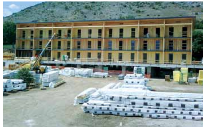
Pre cut walls and partitions are simply brought to site and installed.
