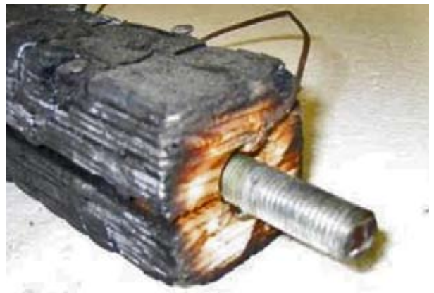
Expoxied rod connection after fire exposure
